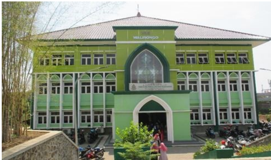
Figure 1. Implementation of glass window and ventilation at Faculty of Psychology and Health
