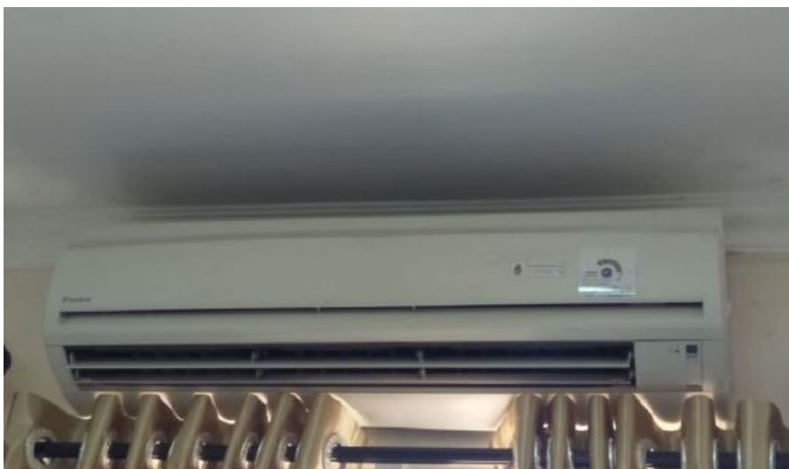
Figure 2. Utilization of Eco-friendly Air Conditioner based smart inverter technology in several building such as Faculty of Psychology and Health building, Faculty of Social Politics building, and Universitas Islam Negeri Walisongo Semarang Office building (Campus 1)
